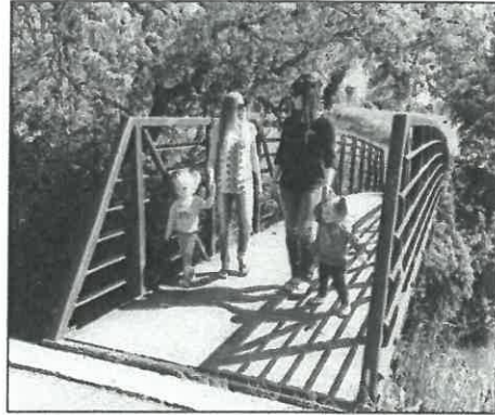
CLAYTON'S WELL-TRAVELED TRAIL BRIDGES received some much needed updating earlier this year. Repairs were funded by the city's Landscape Maintenance District, due to sunset next year. Pictured are Hadley and Julielyn Chippero; Megan and Brooklyn Wahrlich
