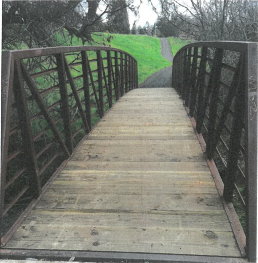
After replacement of wood deck
